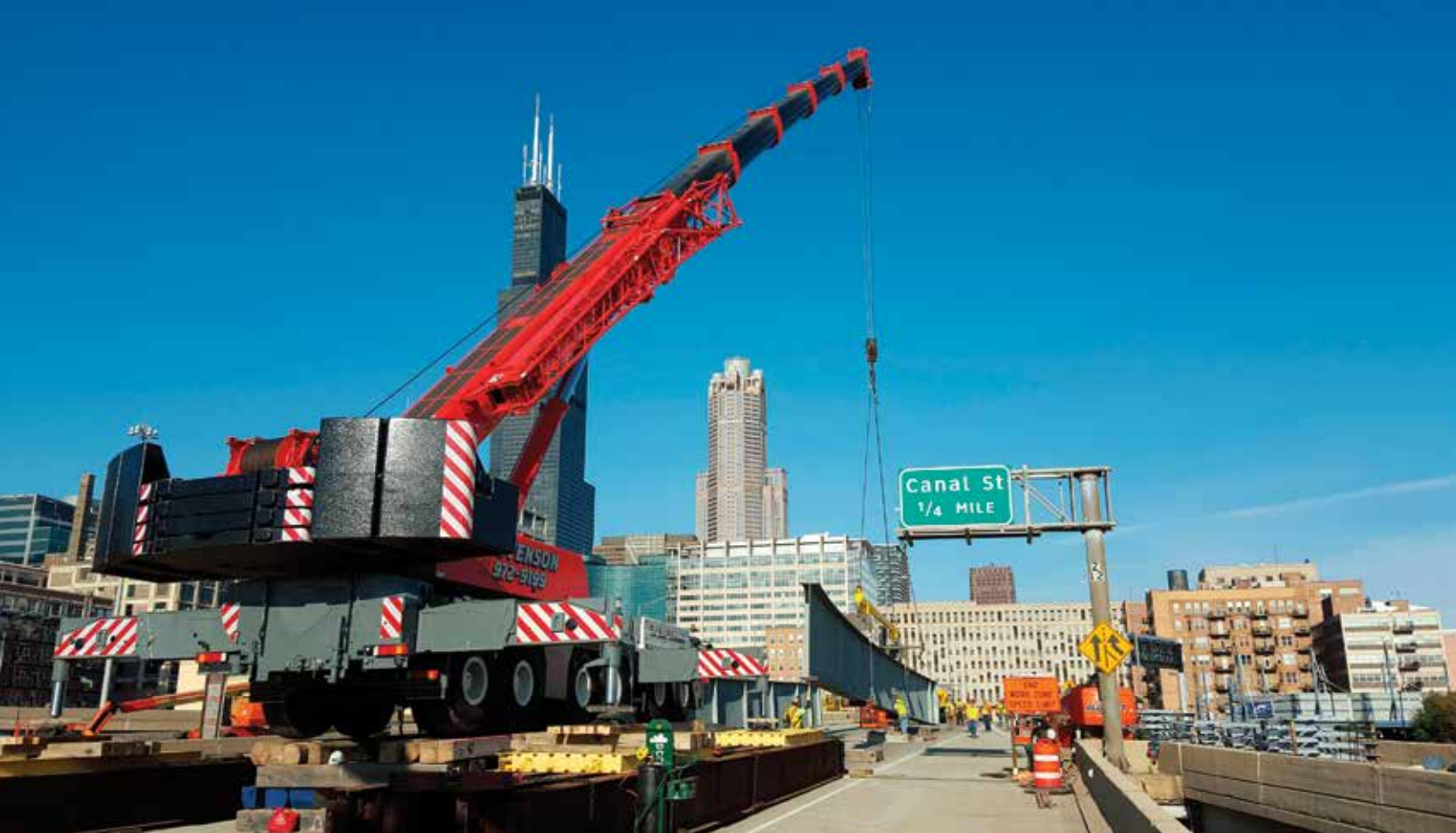
Photo courtesy of Stevenson Crane Service, Inc., Bolingbrook, IL.
