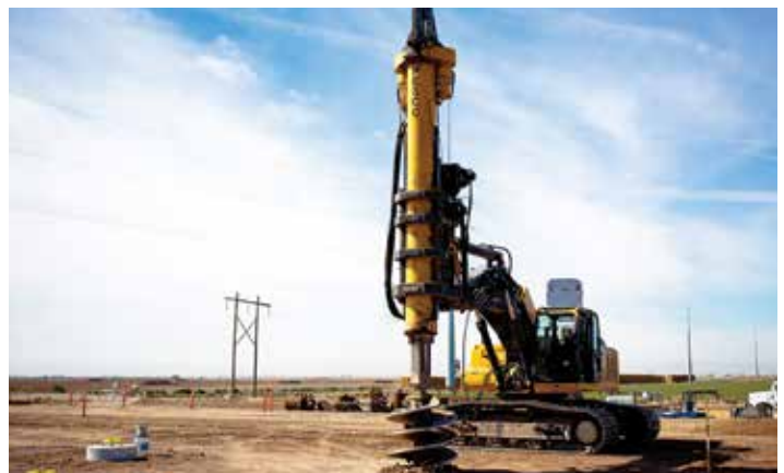
Photo courtesy of Aldridge Electric, Inc., Libertyville, IL.
